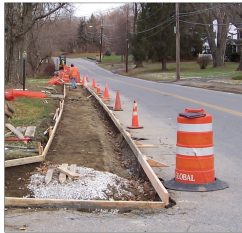
Installation of handicapped accessible sidewalks in the Village of Pawling.
