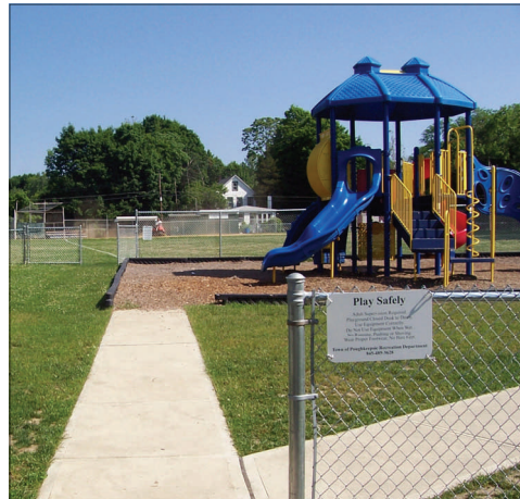
New handicapped accessible playground equipment and walkways in Fairview Park in the Town of Poughkeepsie.
