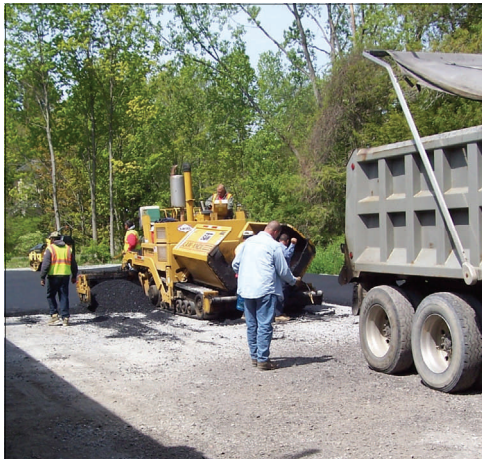
Constructing a new parking lot in the Village of Millerton to create parking for local businesses and the rail trail.
