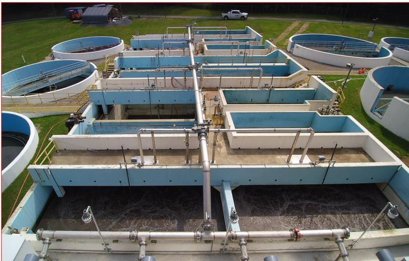
*View of the aeration basins at the Tri-Municipal Wastewater Treatment plant. This system upgrade project was submitted collaboratively by the Village of Wappingers Falls and towns of Poughkeepsie and Wappinger, and was funded in part through the MCSSG program. This new system will increase the plant’s capacity by up to 50% which will allow for future economic development in the vicinity.*
