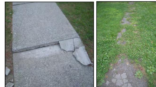
Although most of the sidewalks inventoried were in good or excellent condition, some areas need attention, such as the cracked, settled section on the left, and the disappearing section on the right.
