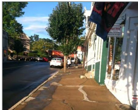
Cracks on Main Street's south sidewalk.
