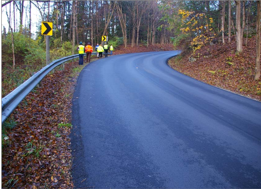
Figure 19. Looking west on Slate Quarry Rd, towards one of two major curves. The outcrop of trees and rocks to the right obscures oncoming vehicles.
