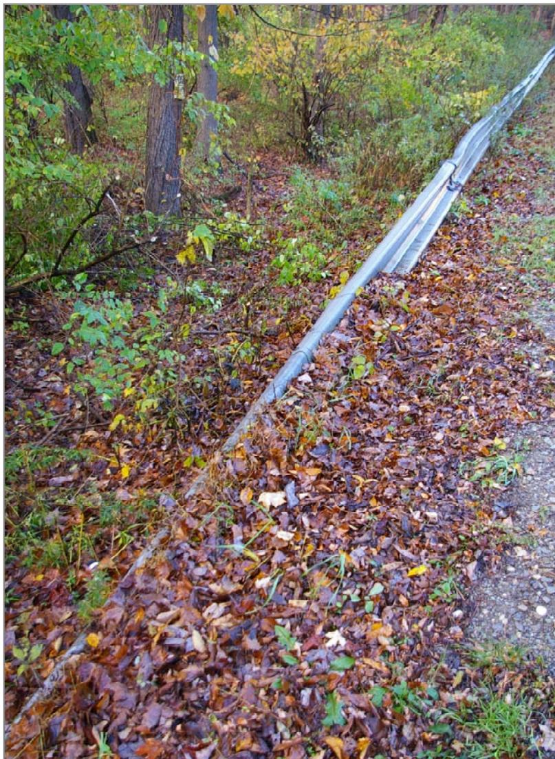
Figure 23. The guidrails along Slate Quarry Rd use the older “W-beam” design, which should be replaced with a “box-beam” design (as shown above on CR16 ). A significant issue with the “W-beam” design involves the end treatment, which can act as a ramp for vehicles that depart the road.
