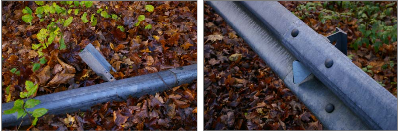
Figure 22. Some of the guidrails along Slate Quarry Rd are in need of repair (left), while delineators should be checked for retro-reflectivity (right).
