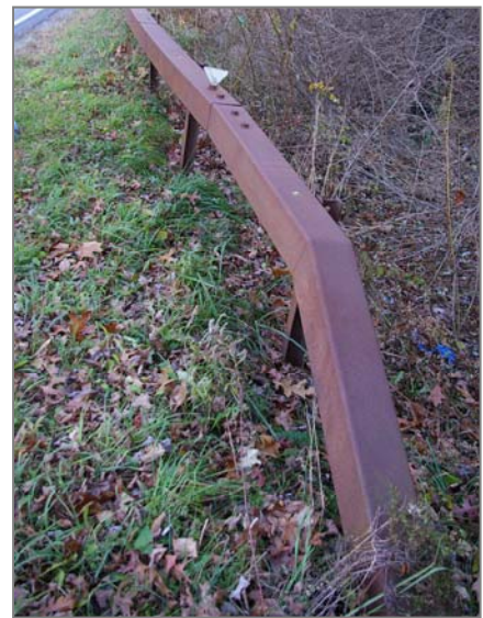
Figure 22. Some of the guidrails along Slate Quarry Rd are in need of repair (left), while delineators should be checked for retro-reflectivity (right).
