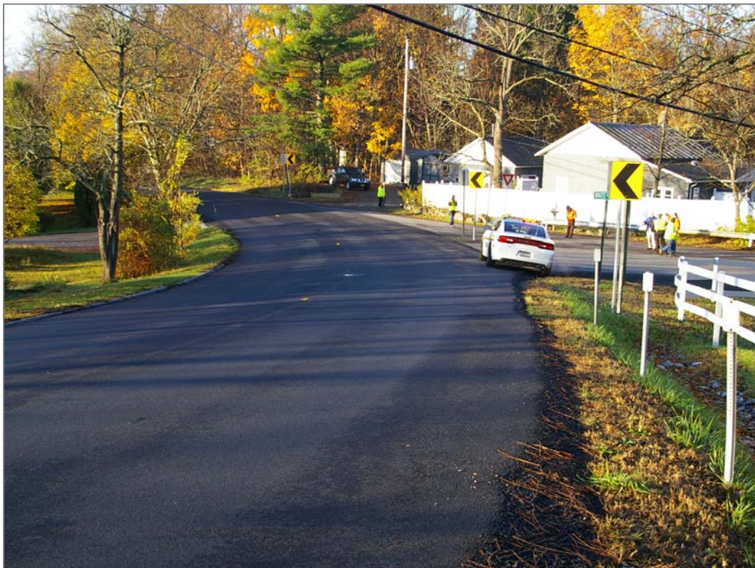
Figure 18. Looking towards White Schoolhouse Rd from westbound Slate Quarry Rd. The trees located to the left, inside the curve, obscure approaching vehicles.
