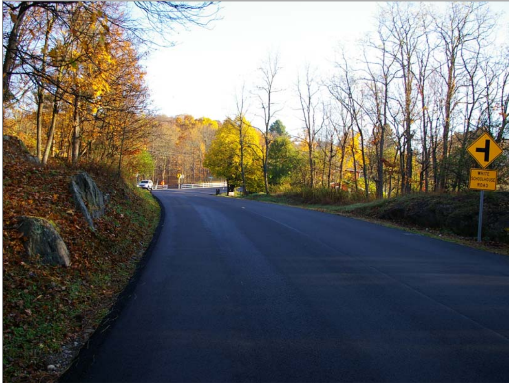
Figure 17. Looking towards White Schoolhouse Rd from eastbound Slate Quarry Rd. Note the change in horizontal geometry towards the curve.
