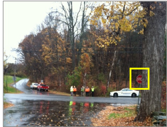
Figure 28. A large tree obscures the STOP sign on the southern approach of Wurtemberg Rd, as it intersects Slate Quarry Rd.
