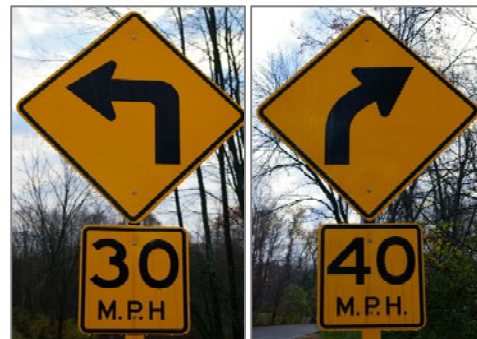
Figure 21. A variety of advisory speeds are used along Slate Quarry Rd.
