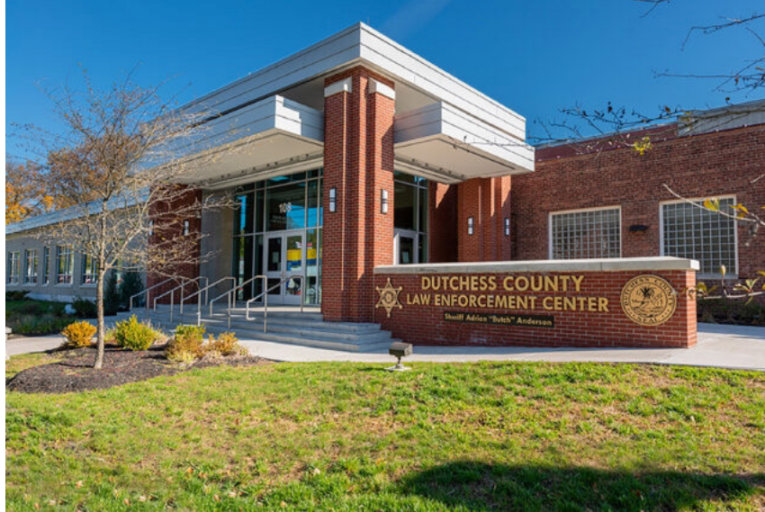
Completed LEC as of Summer 2019.
