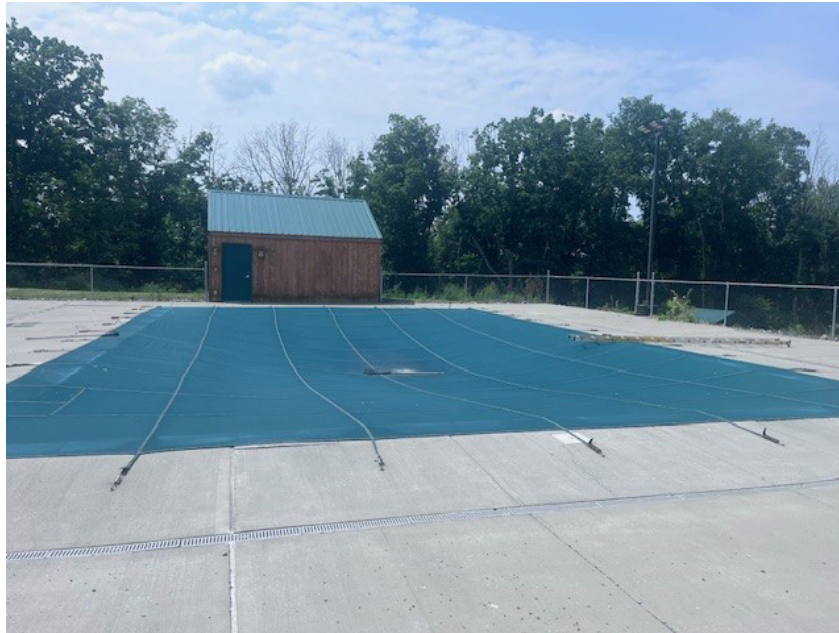
Partially completed pool at Camp Nooteeing with safety pool covering.
