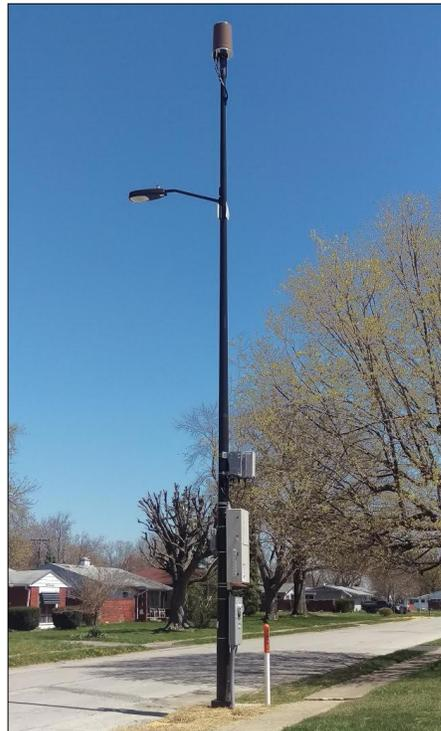
*On the left, a new pole holding small cell equipment installed in the right-of-way in Albany, NY. On the right, an example of a small cell integrated into a municipal streetlight. (Photo Credits: Paula Gilbert (l), NYS DOS (r))*
