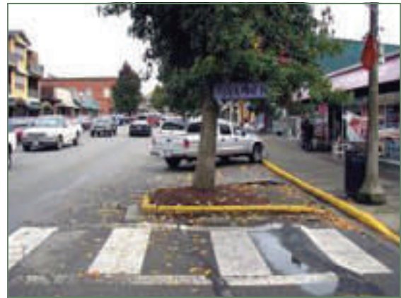
This tree well in the parking lane calms traffic and protects the crosswalk. Photo credit: FHWA.
