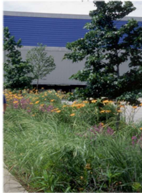
Bio-retention filter could be required to address exceeding lot coverage for parking
