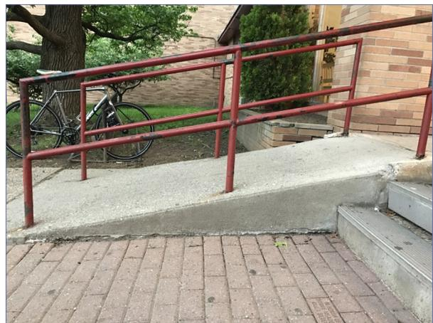
*Ramps are only positive tools for accessibility when constructed to the appropriate standards. Participants were hard-pressed to either go up or down this steep ramp in a wheelchair.*
