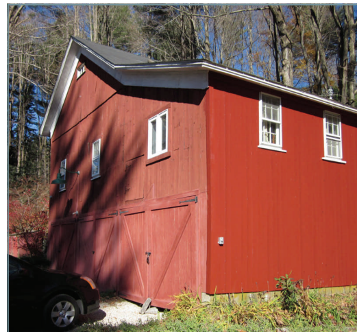
Though not obvious from the outside, this barn in Cornwall, CT has been converted into an accessory dwelling unit.
