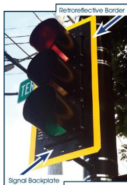
Backplates with Retro-reflective Borders (source: FHWA)
