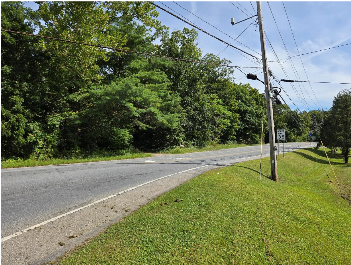
Pine Woods Rd in Hyde Park, which was a Field Investigation site and is a focus facility for Roadway Departure Crashes, is an example of where a roadway departure could lead a vehicle down a roadside slope.
