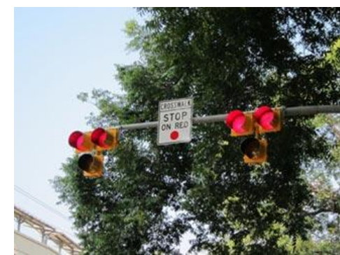
Pedestrian Hybrid Beacon (PHB) (source: FHWA)
