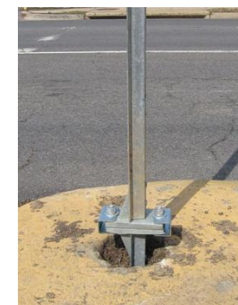
Breakaway Sign Supports (source: FHWA)
