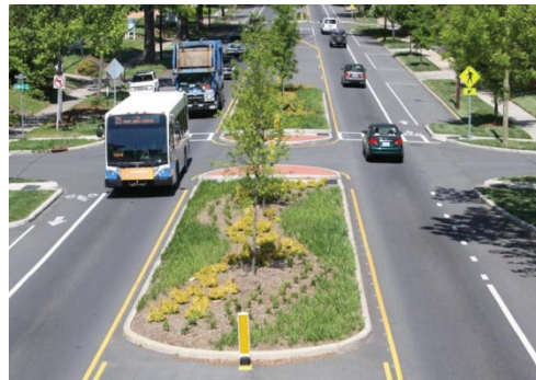
Median Island (source: FHWA)
