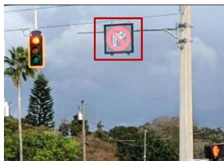
No Turn on Red Sign (Overhead Blank-Out –) (source: CUTR)
