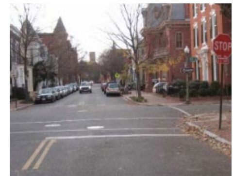
Painted Stop Bar (source: FHWA)
