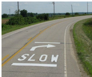
Curve Warning Pavement Markings (source: Iowa Center for Transportation Research and Education)
