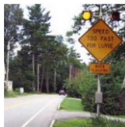
Flashing Beacons on Warning Signs (source: FHWA)
