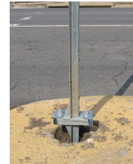
Breakaway Sign Supports (source: FHWA)
