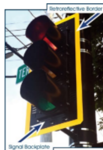
Backplates with Retro-reflective Borders (source: FHWA)
