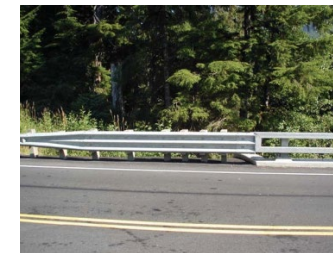
Roadside Barriers (source: FHWA)
