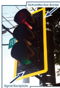
Backplates with Retro-reflective Borders (source: FHWA)
