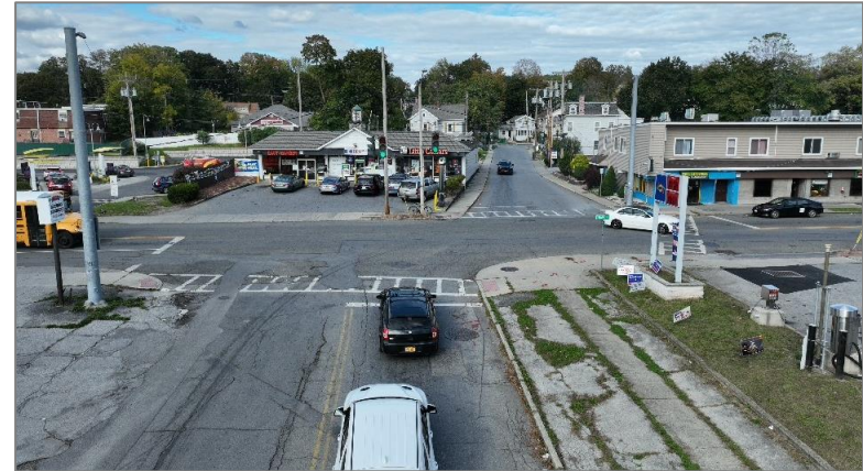
We continued to work with County Public Works in progressing several transportation initiatives, including redesigning the Main St/Grand Ave intersection in the Town of Poughkeepsie.
