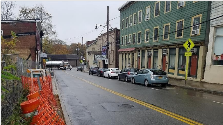
Large trucks can find it difficult to navigate the narrow dimensions of Route 9D as it travels through Wappingers Falls above. We looked at this and other issues along the 9D corridor.
