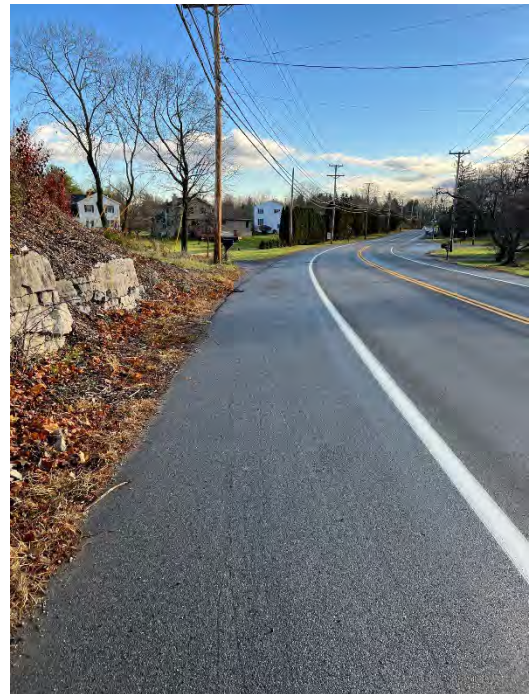
Existing wide shoulder on Spackenkill Rd
