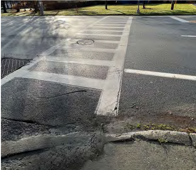
Croft Rd crosswalk
