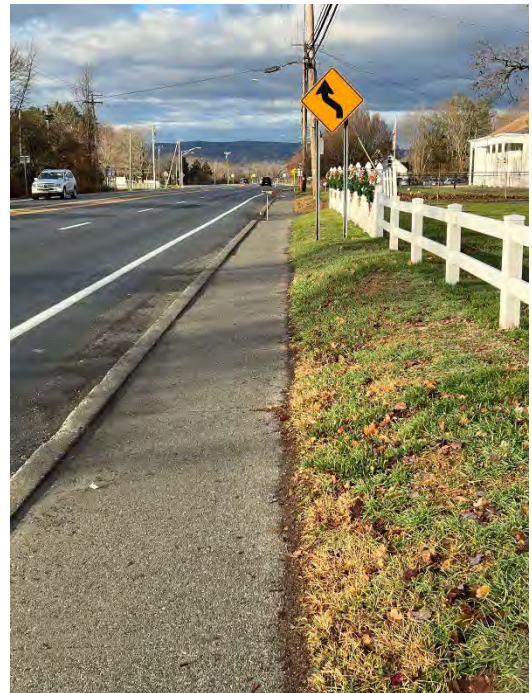
Existing sidewalk on Spackenkill Rd, west of study area
