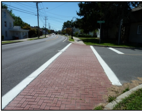
Stamped, well-marked crosswalks in Port Ewen, NY are aesthetically pleasing and provide a strong visual cue to drivers that they should be on the lookout for pedestrians.
