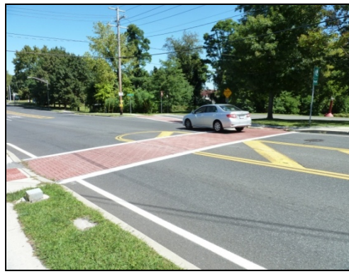
Stamped, well-marked crosswalks in Port Ewen, NY are aesthetically pleasing and provide a strong visual cue to drivers that they should be on the lookout for pedestrians.
