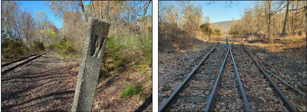
Figure 2: “W” Post (left) and railroad switch (right).
