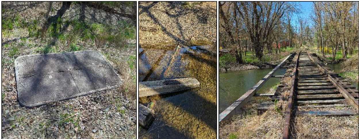
Figure 11: Metro-North fiber optic pullbox (left), exposed fiber-optic conduit from a washout (middle), and conduit hanger on Bridge #5 (right).
