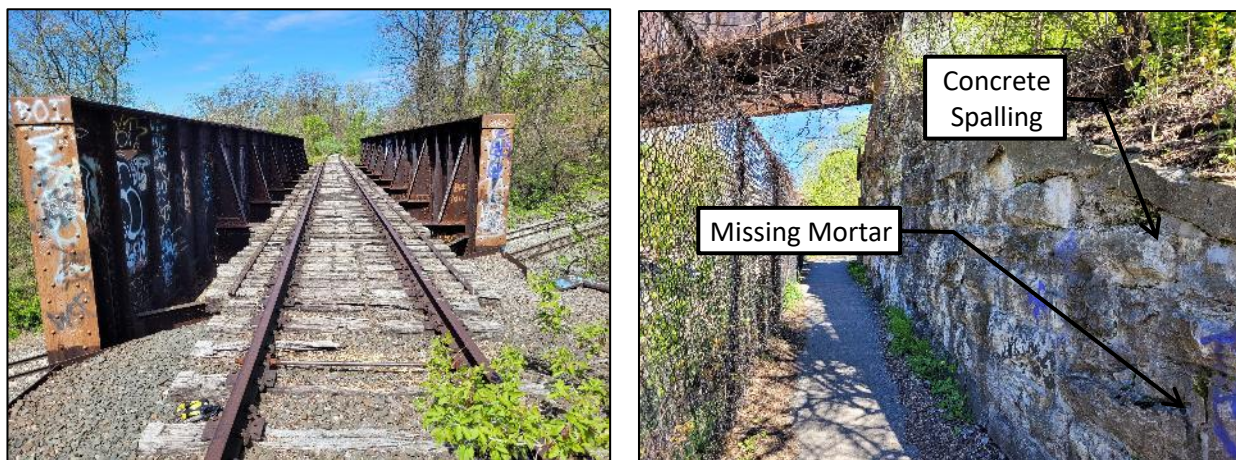
Figure 20: Bridge No. 1 through girder superstructure (left) and stone masonry substructures (right).
