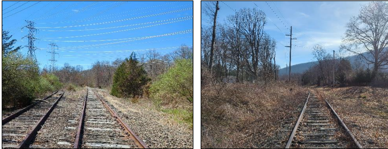
Figure 12: Overhead electric transmission lines near the CHG&E sub-station (left) and overhead electric transmission lines east of Washington Ave (right).
