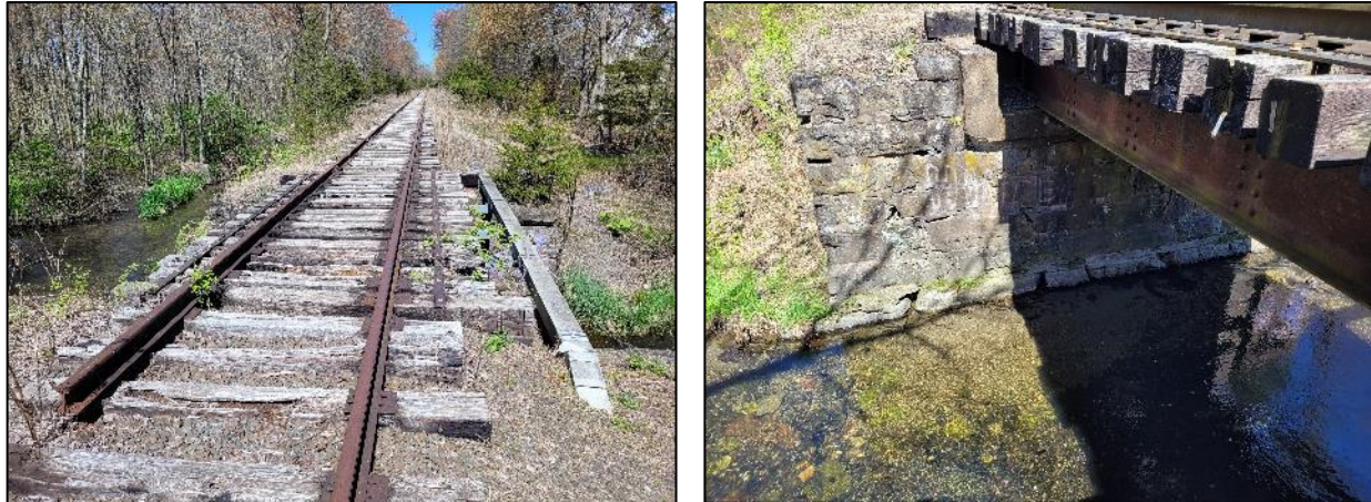
Figure 29: Bridge No. 6 superstructure (left) and substructure (abutment and wingwall) (right).
