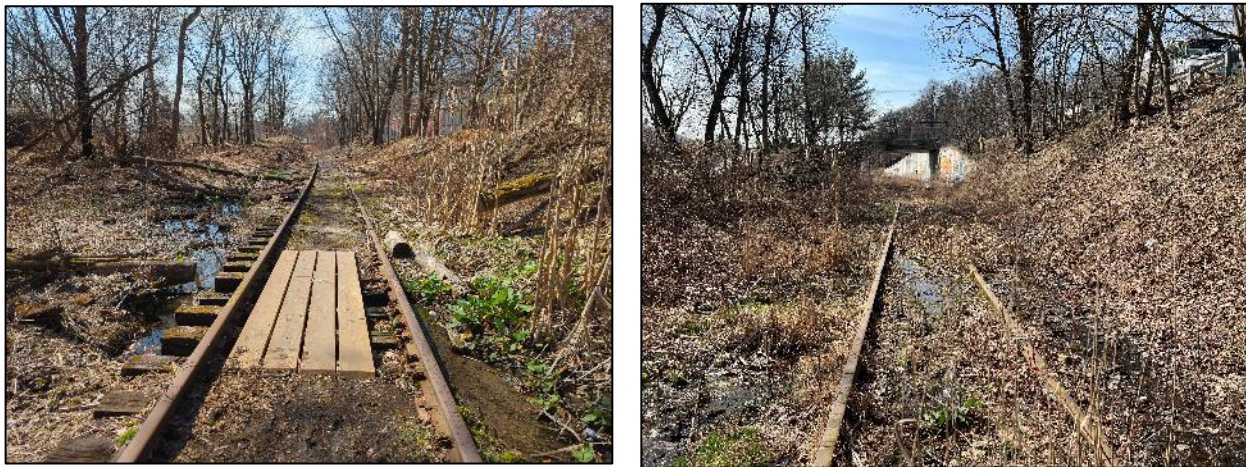
Figure 8: Uncontrolled stream crossing 500 feet east of Main Street (left) and possible wetland area 300 feet east of the Route 9D (Wolcott Ave) overpass.
