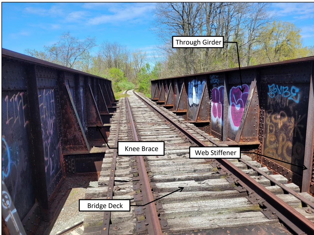
Figure 18: Through Girder Bridge Components.
