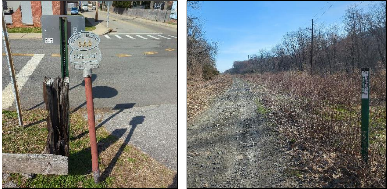
Figure 10: An underground gas pipeline marker along Main St. in the City of Beacon (left) and overhead electric transmission lines and a sewer pipeline marker east of Washington Ave (right).
