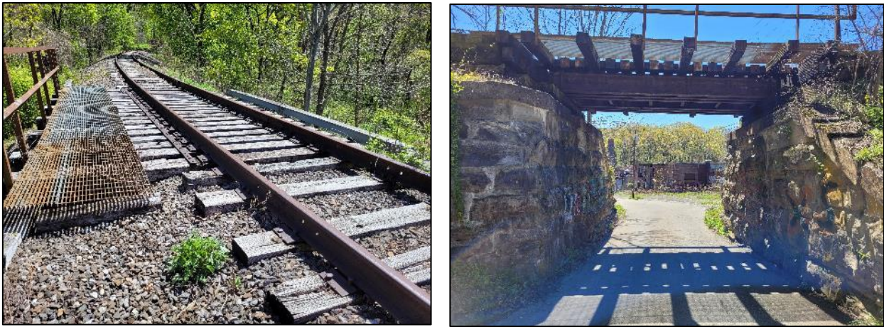
Figure 21: Bridge No. 2 superstructure (left) and stone masonry substructures (right).
