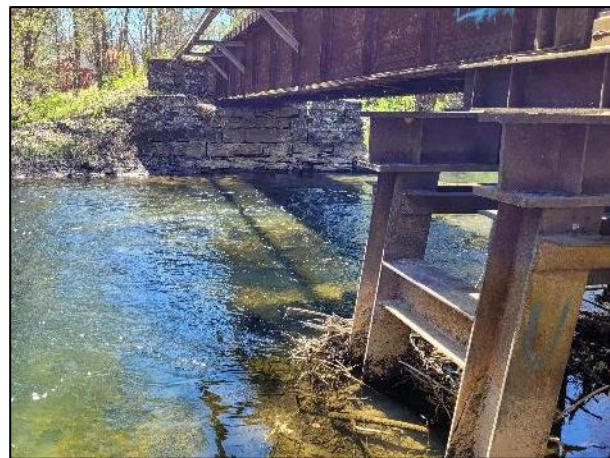
Figure 27: Bridge No. 5 superstructure (left) and stone masonry abutment and pile bent substructures (right).
