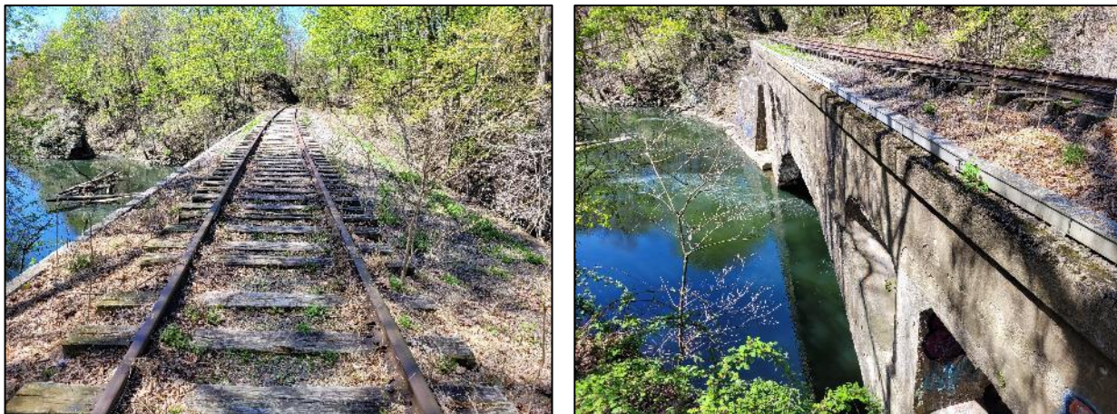
Figure 23: Bridge No. 3 superstructure (left) and concrete spandrel arch substructures (right).
